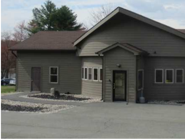
Clubhouse siding overview
