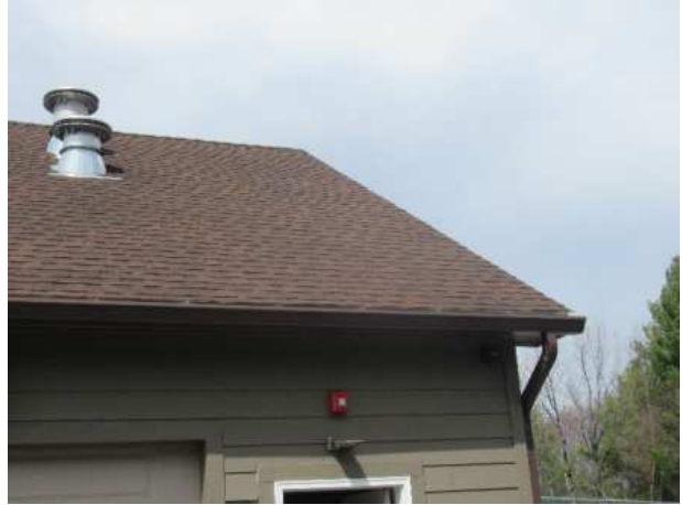
Pool mechanical building roof overview
