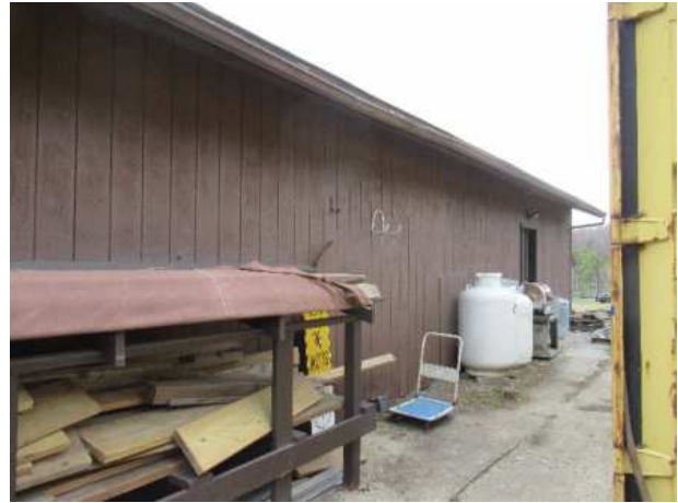
Wood siding at the maintenance building
