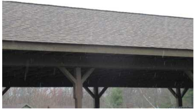
Asphalt shingle roof overview
