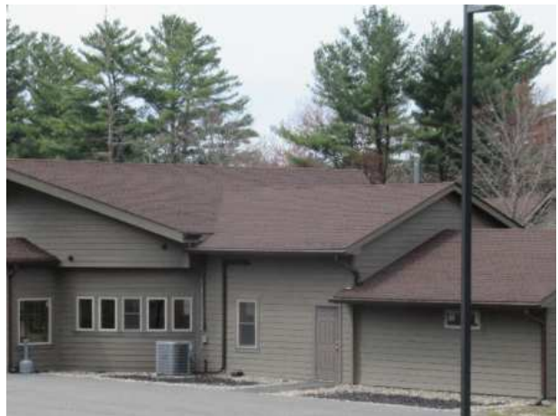
Clubhouse roof overview
