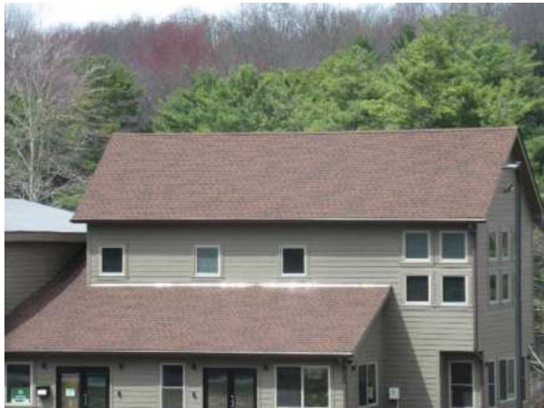
Entertainium building roof overview
