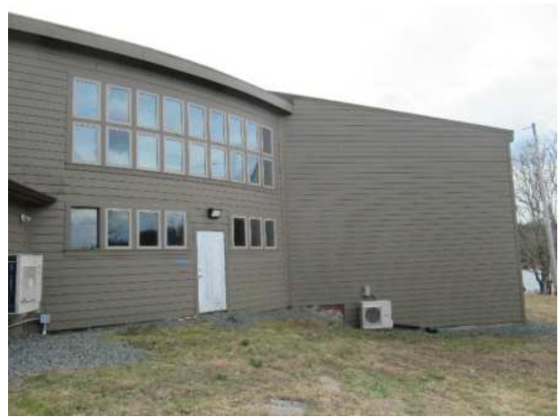
Siding overview at the entertainium building
