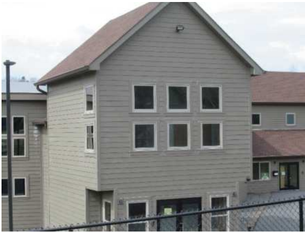
Siding overview at the entertainium building
