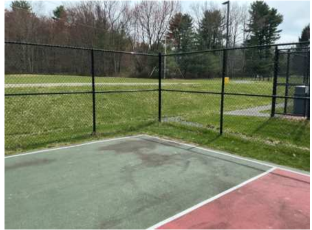
Basketball fence overview
