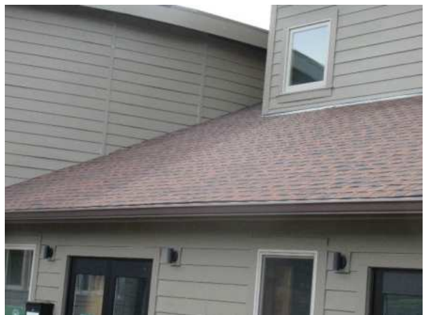
Entertainium building roof overview
