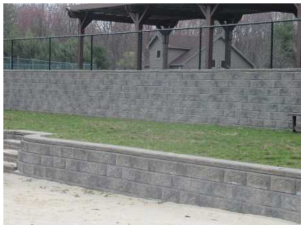
Masonry walls at the pool house and beach
