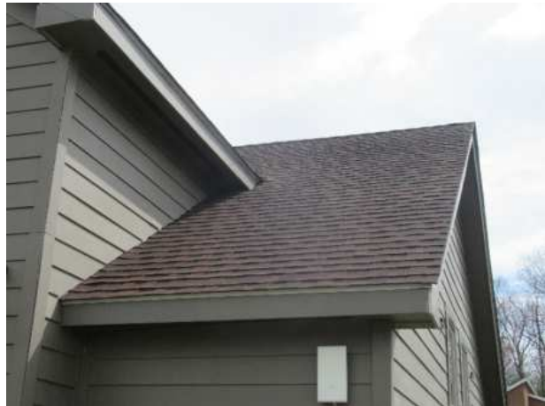
Pool mechanical building roof overview
