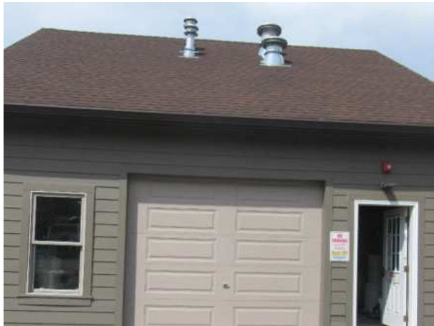
Pool mechanical building roof overview
