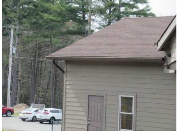
Clubhouse roof overview
