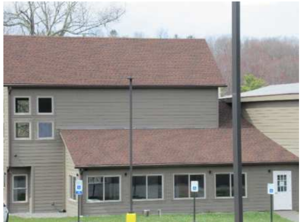
Entertainium building roof overview
