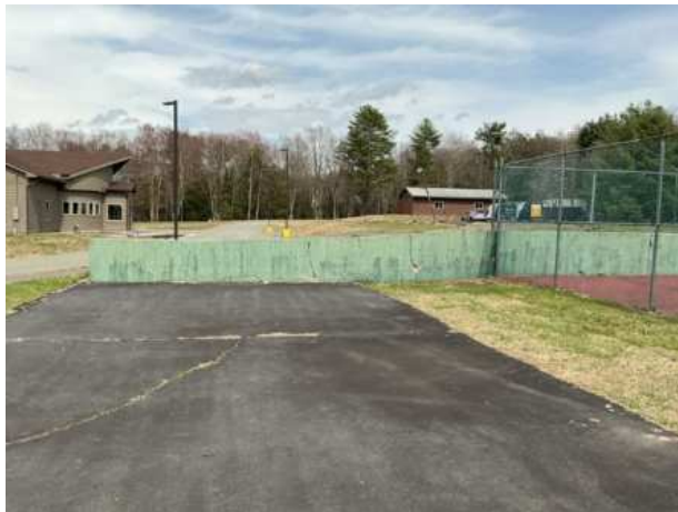
Concrete retaining wall
