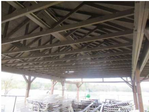
Pavilion structure detail
