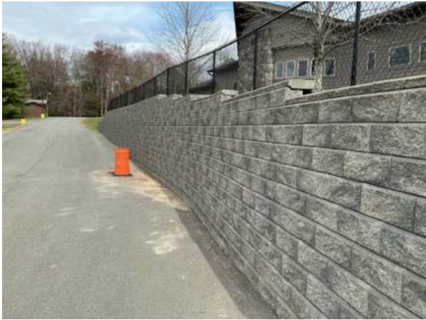
Masonry wall at the clubhouse
