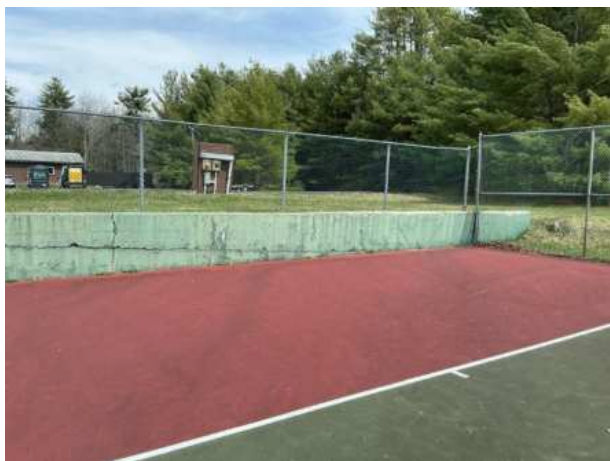
Concrete retaining wall
