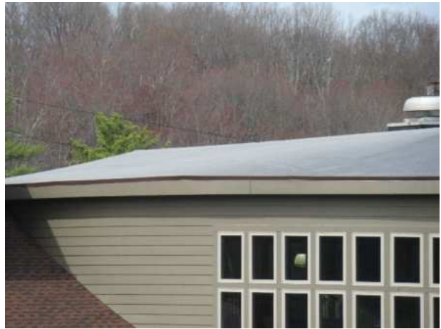
EPDM roof overview
