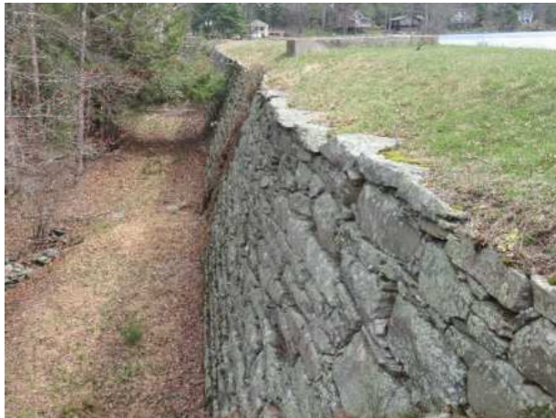
Earthen dam at Lake Louise Marie
