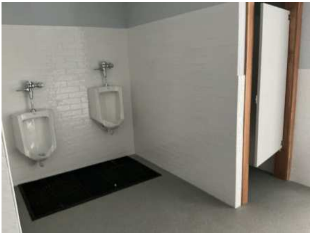
Pool house locker room overview
