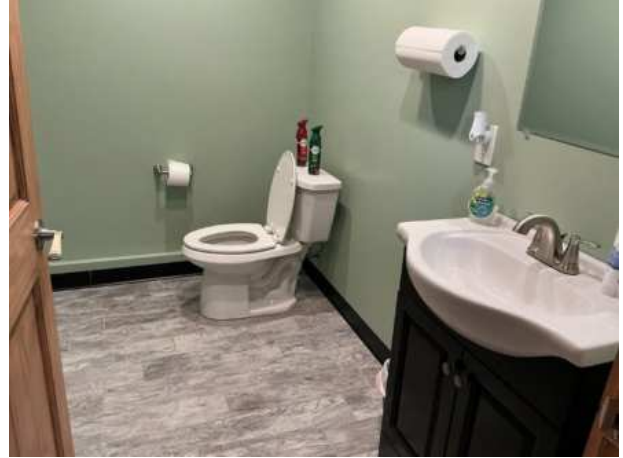
Rest room overview
