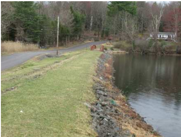
Earthen dam at Lake Davies
