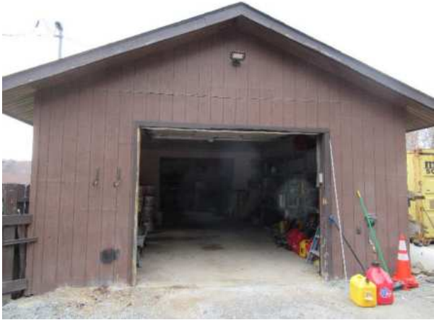
Wood siding at the maintenance building
