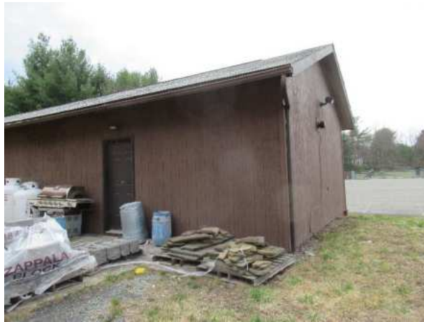
Wood siding at the maintenance building
