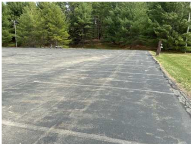
Upper parking area near clubhouse
