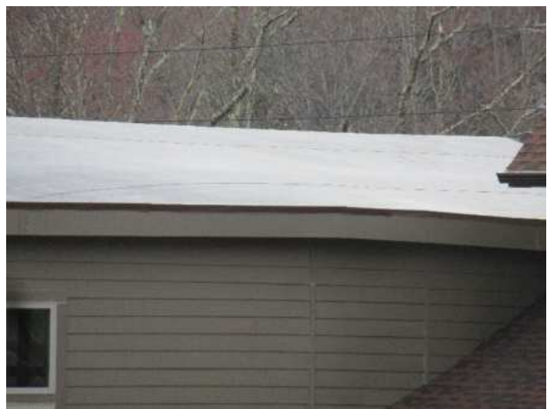
EPDM roof overview
