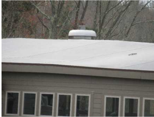
EPDM roof overview
