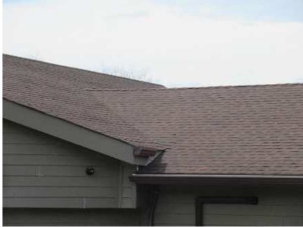
Clubhouse roof overview
