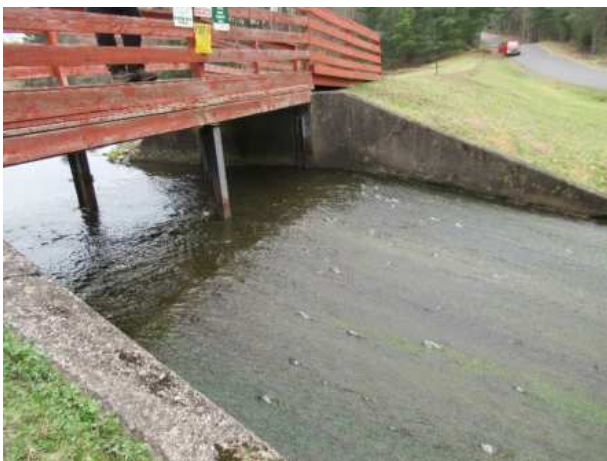
Concrete spillway at Lake Davies
