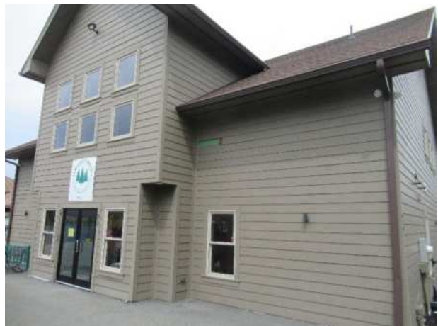
Pool house siding overview
