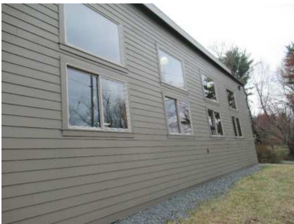
Siding overview at the entertainium building
