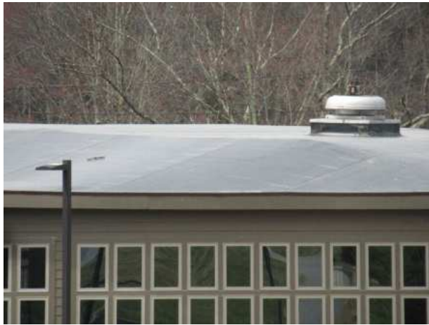
EPDM roof overview
