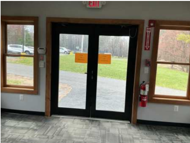
Windows and Doors
