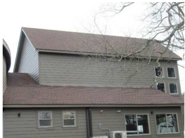
Siding overview at the entertainium building
