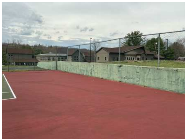
Concrete retaining wall
