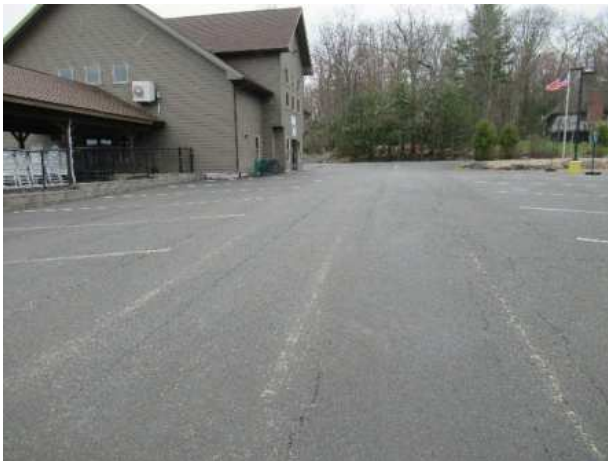
Pool house parking area overview
