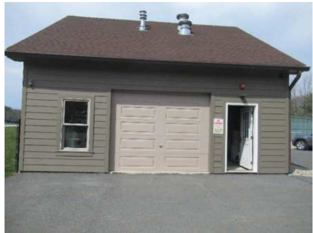
Pool mechanical building rear
