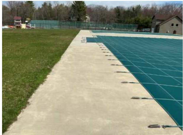
Concrete deck overview
