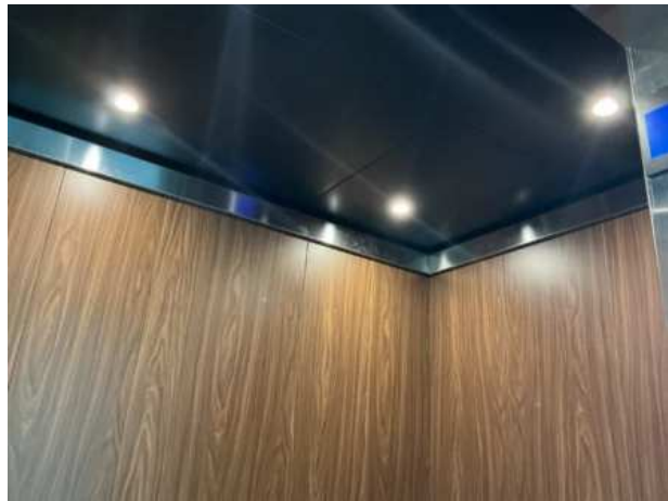
Wood panel walls and metal ceiling coverings
