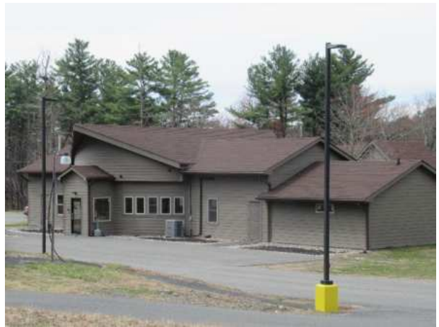
Light poles and fixtures near the clubhouse
