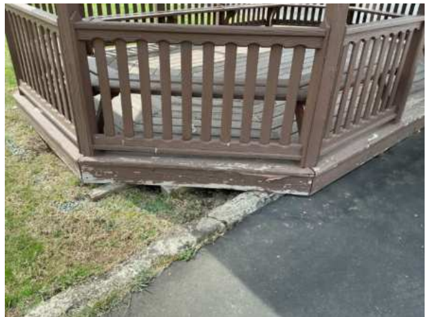
Finish deterioration
