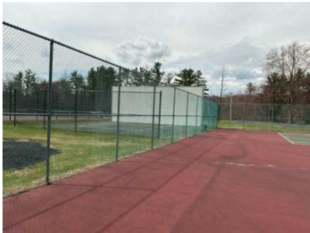
Tennis court fence at the clubhouse
