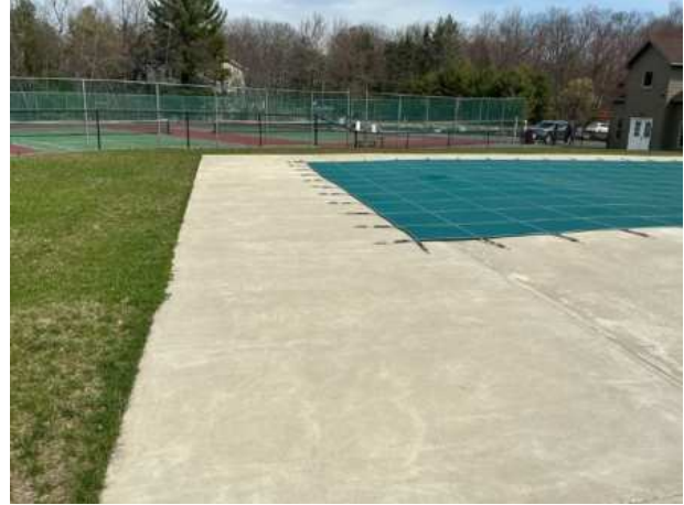
Concrete deck overview
