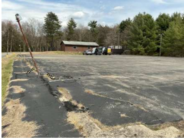
Upper parking area near clubhouse
