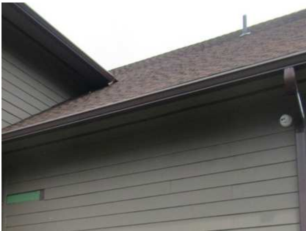
Pool house roof overview
