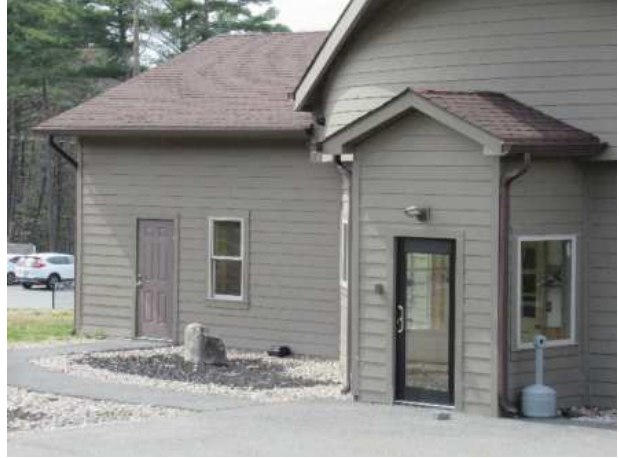
Clubhouse siding overview
