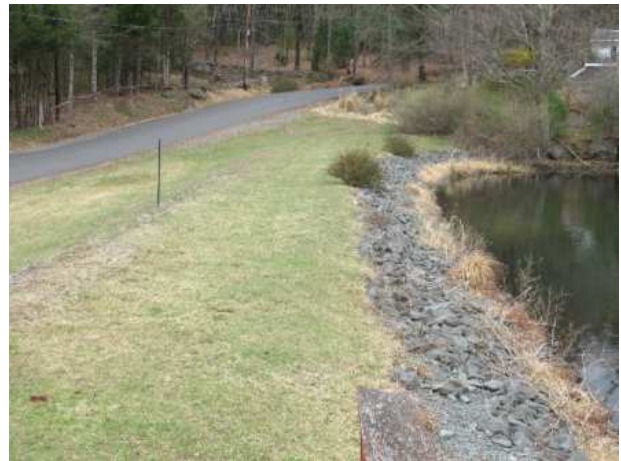
Earthen dam at Lake Davies
