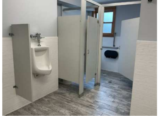
Locker room overview
