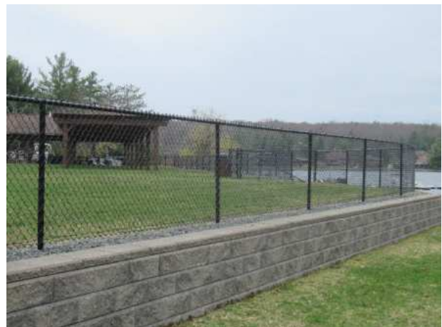
Chain link fence
