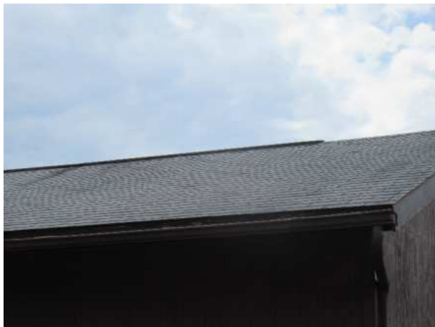
Maintenance building roof overview
