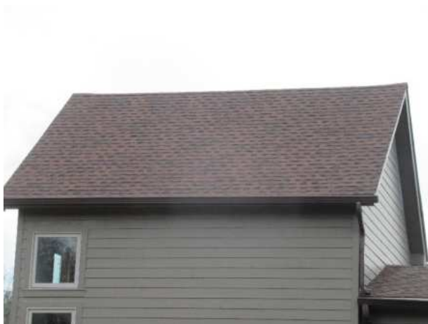
Entertainium building roof overview
