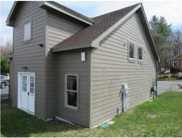
Pool mechanical building siding overview
