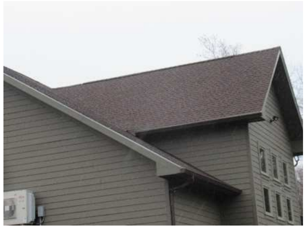
Pool house roof overview
