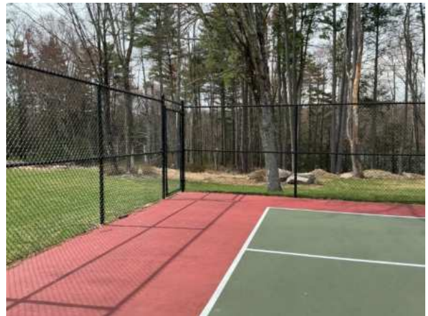
Pickleball fence overview
