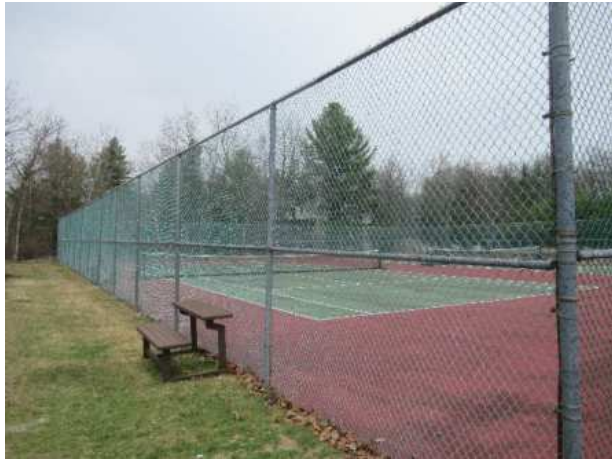
Tennis court fence at the pool house
