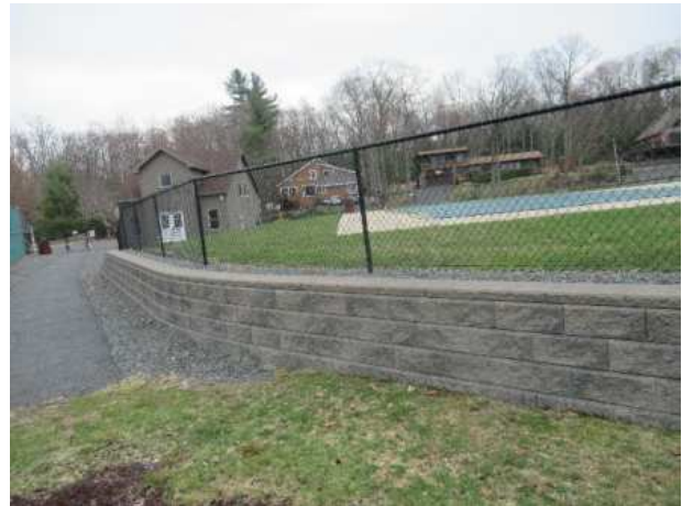
Chain link fence
