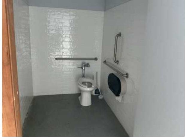
Pool house locker room overview
