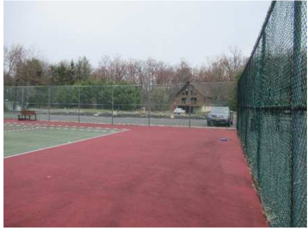
Tennis court fence at the pool house
