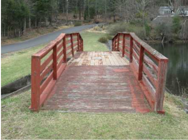
Wood bridge overview
