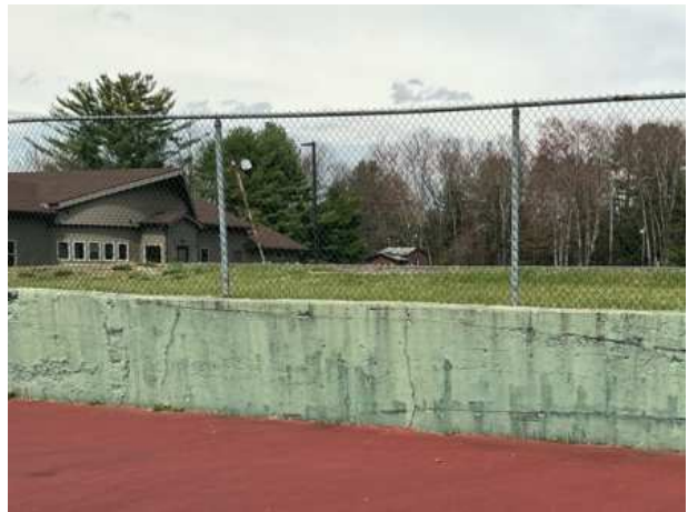
Tennis court fence at the clubhouse
