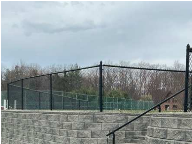
Chain link fence
