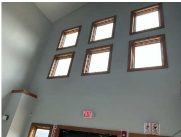
Pool house interior overview
