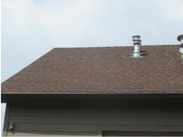
Pool mechanical building roof overview
