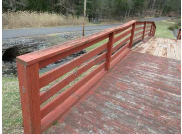
Wood bridge overview
