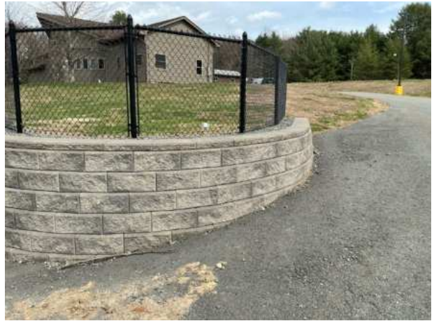
Masonry wall at the clubhouse
