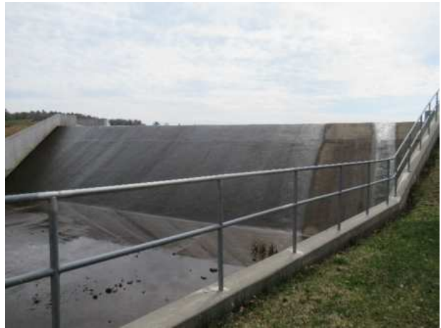
Concrete spillway at Lake Louise Marie
