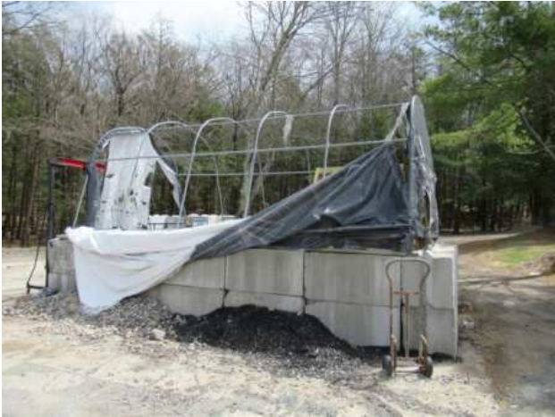
Salt Storage Area
