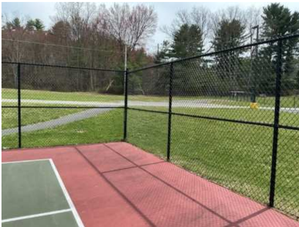
Pickleball fence overview
