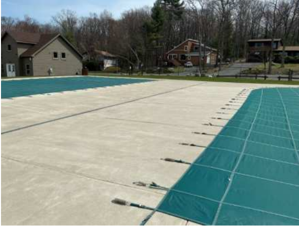
Concrete deck overview
