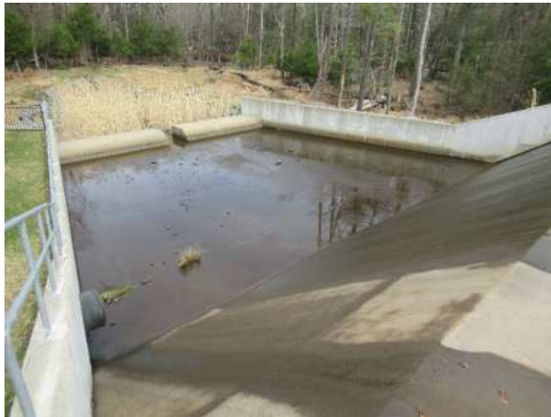
Concrete spillway at Lake Louise Marie
