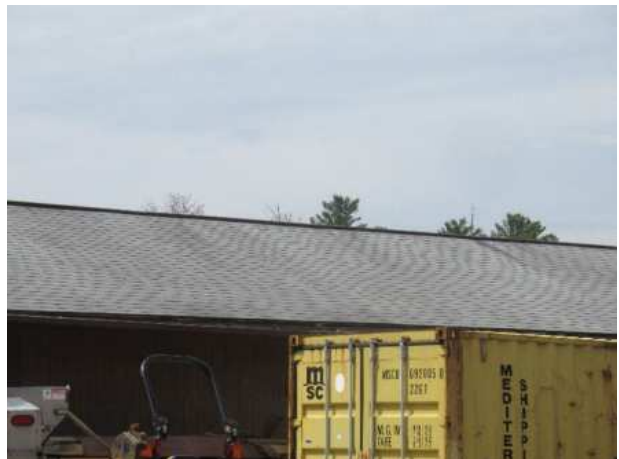
Maintenance building roof overview
