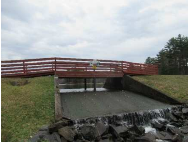
Concrete spillway at Lake Davies
