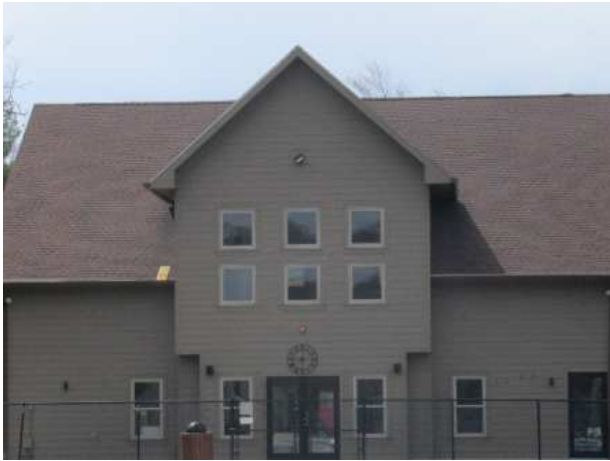
Pool house roof overview
