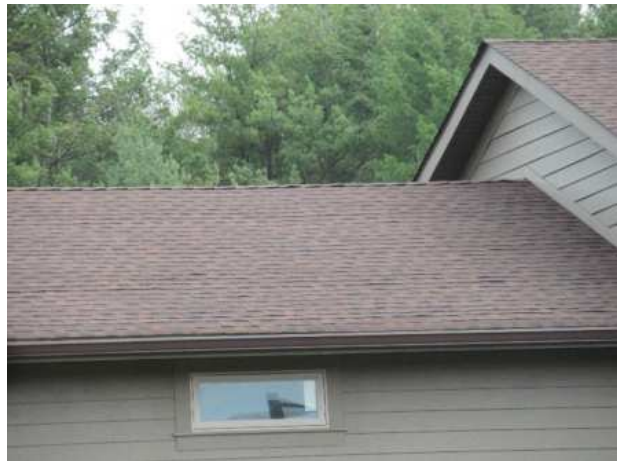
Shingle lift at the clubhouse
