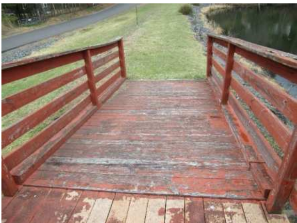
Finish deterioration
