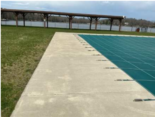
Concrete deck overview
