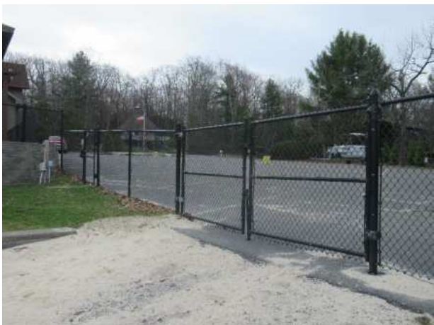
Chain link fence
