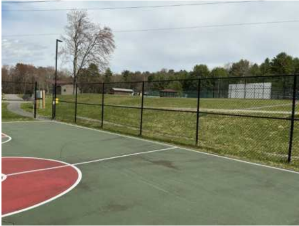
Basketball fence overview
