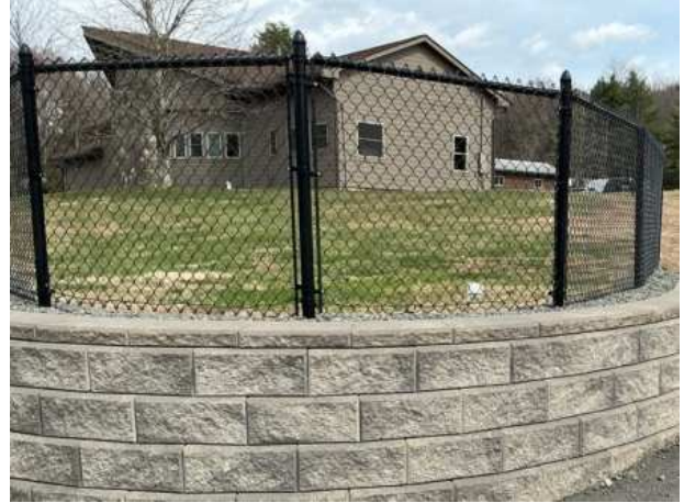
Chain link fence on top of the masonry wall
